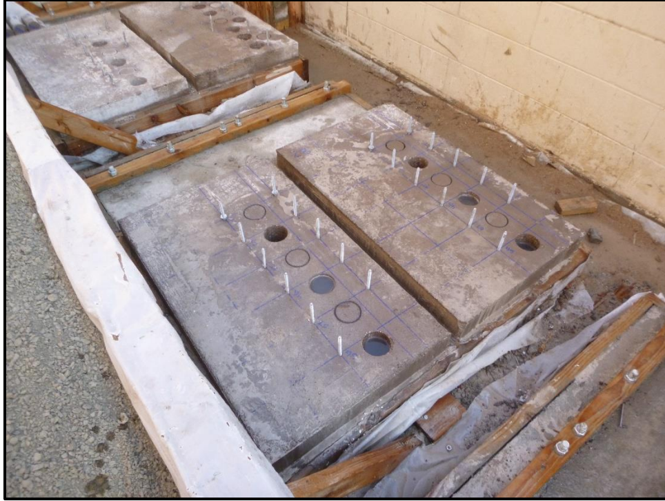
Figure 3-8 – As constructed view showing pull-off test sampling locations.
