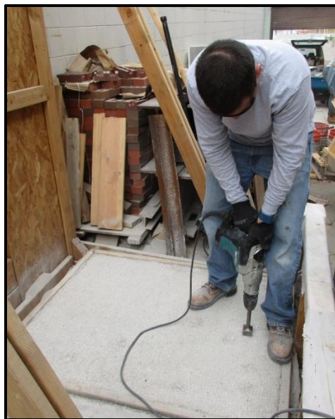
Figure 3-2 – Surface profiling the substrate
