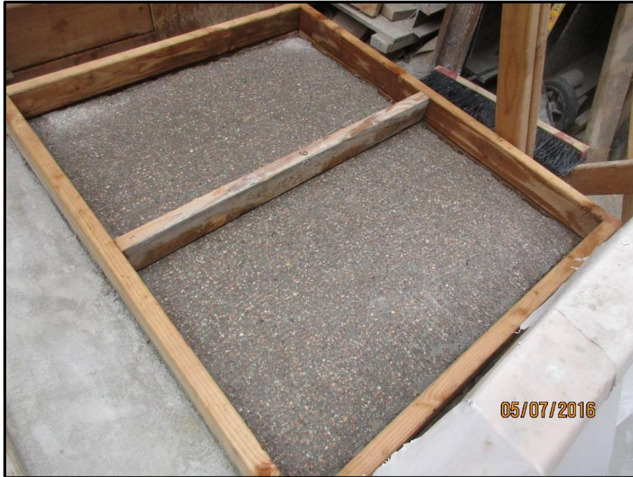
Figure 3-4 – Example of saturated, surface dry appearance immediately before placement
