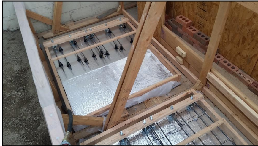
Figure 3-1 – Typical substrate form, ready to receive concrete
