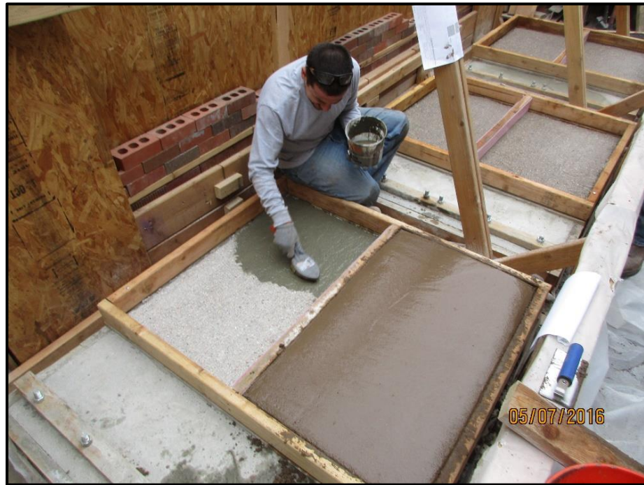
Figure 3-5 – Application of cement slurry bonding agent
